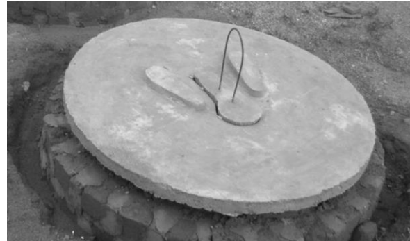
A cement slab with lid and raised foot rests. Ready for construction of the latrine walls
